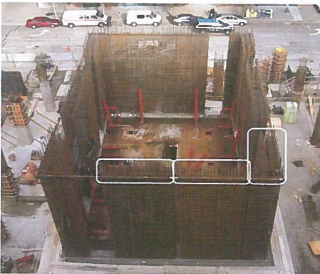
Figure 6.32 Pre-Tied Modules (Some Modules Encircled).
