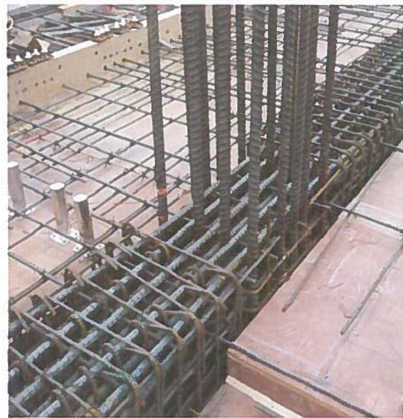
Figure 6.20 Beam-Column Joint with Small Diameter Corner Bars
