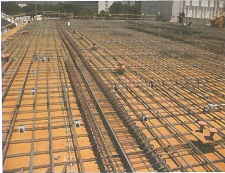
Figure 6.48 A Long Collector with Confinement Reinforcement.
