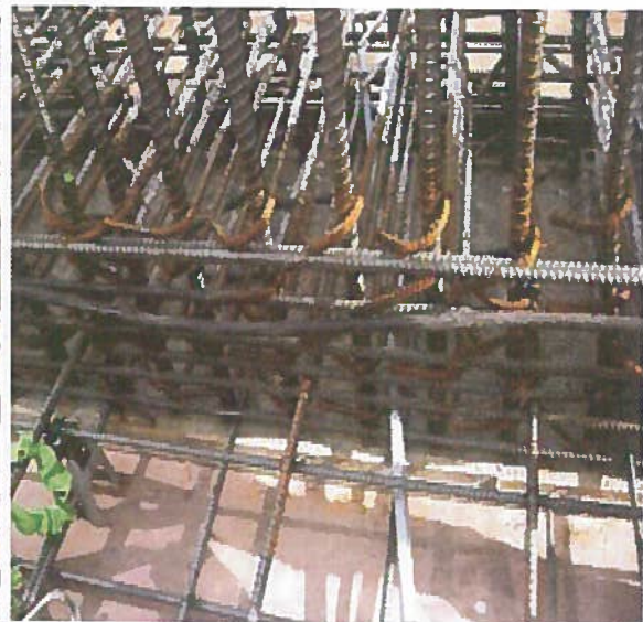
Figure 6.33 Boundary Confinement for Planar Wall
