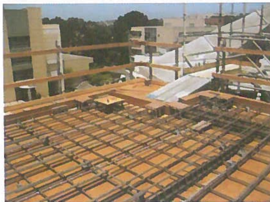
Figure 6.49 Confinement of a Collector.
