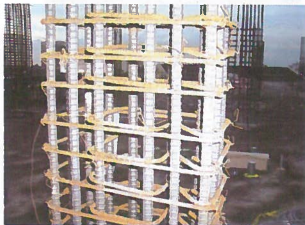
Figure 6.22 Column Cage with Hoops Constructed from Single Reinforcing Bar.
