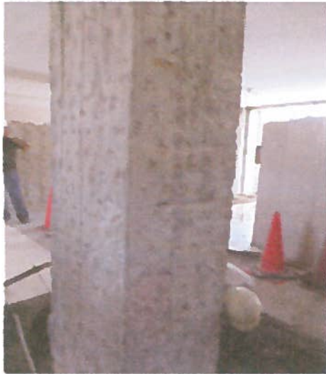
Preparation of Column Steel Jacking in a School at Chiba City
