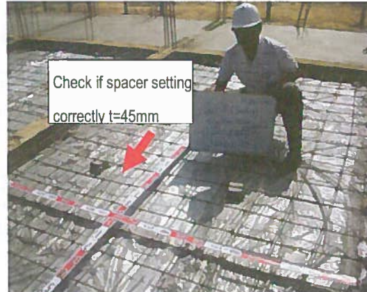
PHOTO 2: Check size of bar D6, pitches @ 200mm, overlap 270 mm
