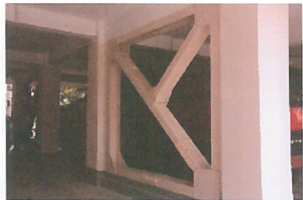
Internal Steel Frame Bracing after construction
