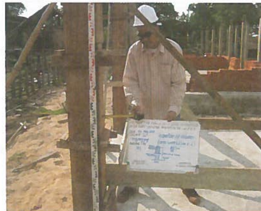
PHOTO 4: Checking verticality of formwork by plumbing
