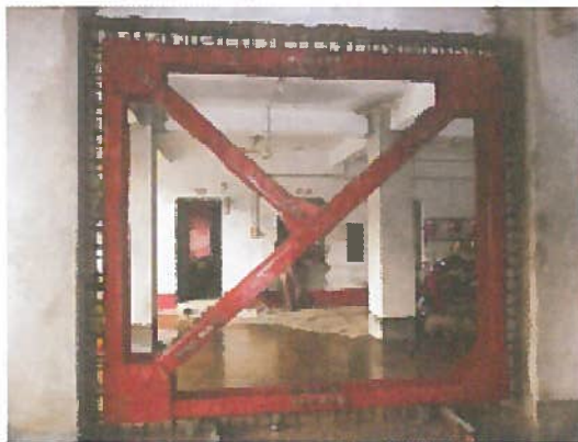
Internal Steel Frame Bracing under construction
