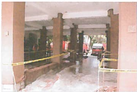
Photos of RC column jacking
