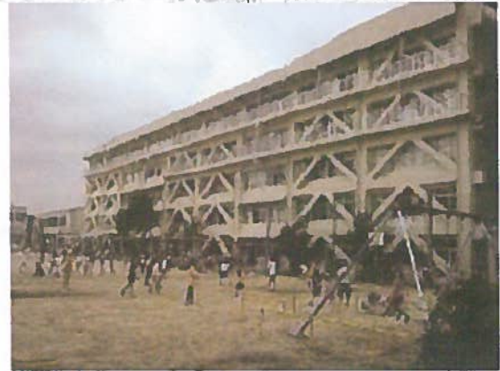
d) Elementary School Building (with Balconies)
