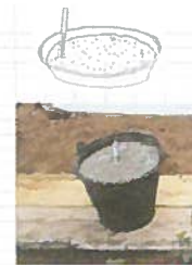
Concrete temperature check
