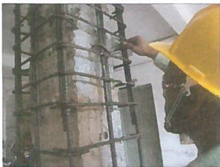
Chemical Applying on old Column Surface
