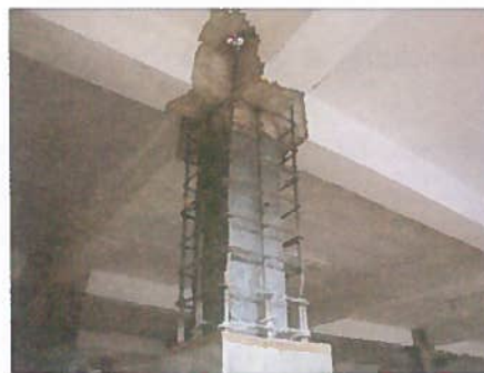
Column Jacking Work at site
