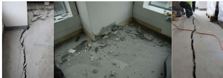
(b) Loss of Strut Landing Points Due to Significant Perimeter Cracking (Fenwick et al. 2010)
