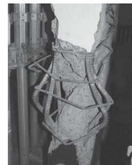
(b) Inadequately detailed transverse reinforcement at wall boundary
