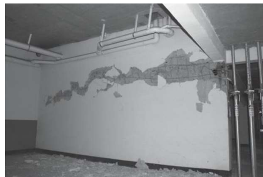
(a) Overall view of crushed wall
